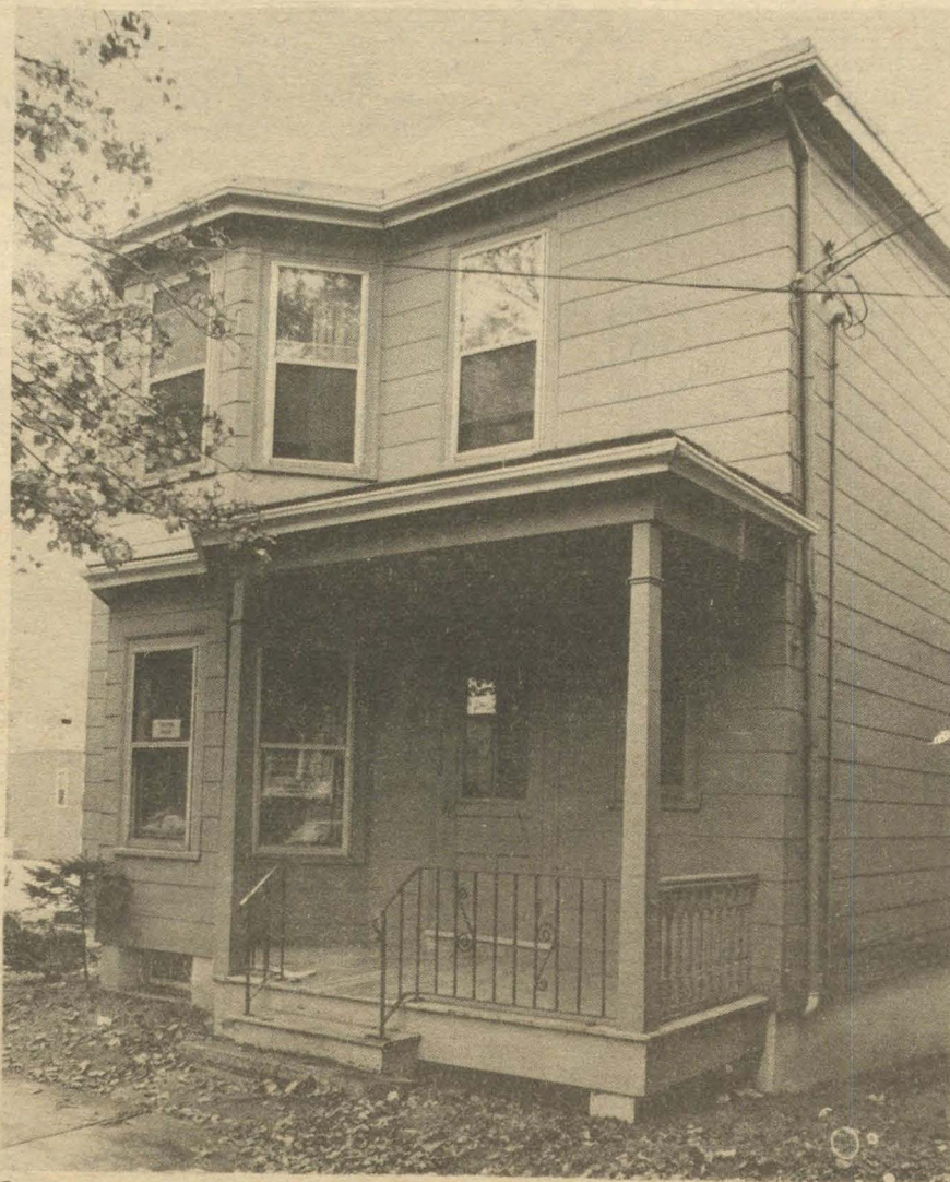
Students of Dalhousie's lower campus find fleeting happiness in Carleton House. The house, newly renovated, is soon to be taken away.
