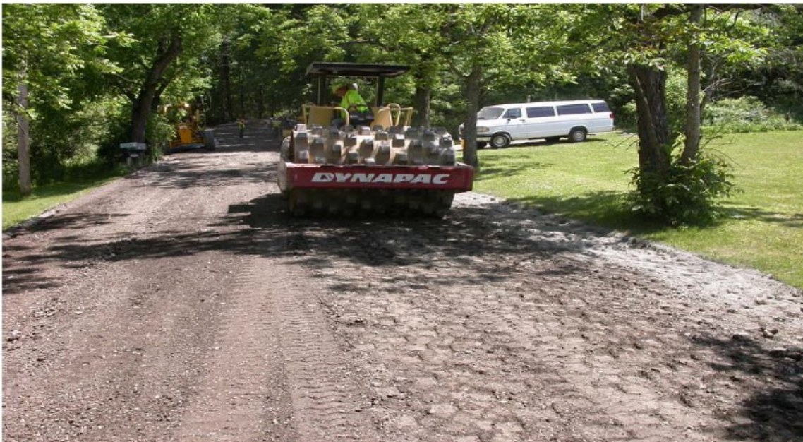
Figure 2-5 Compacting the pavement with a sheep's foot roller (Morian et al., 2012)
