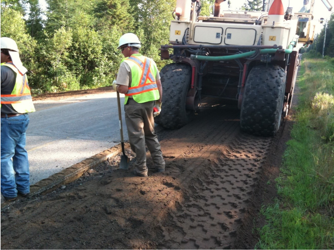
Figure 2-7 FDR process in existing pavement
