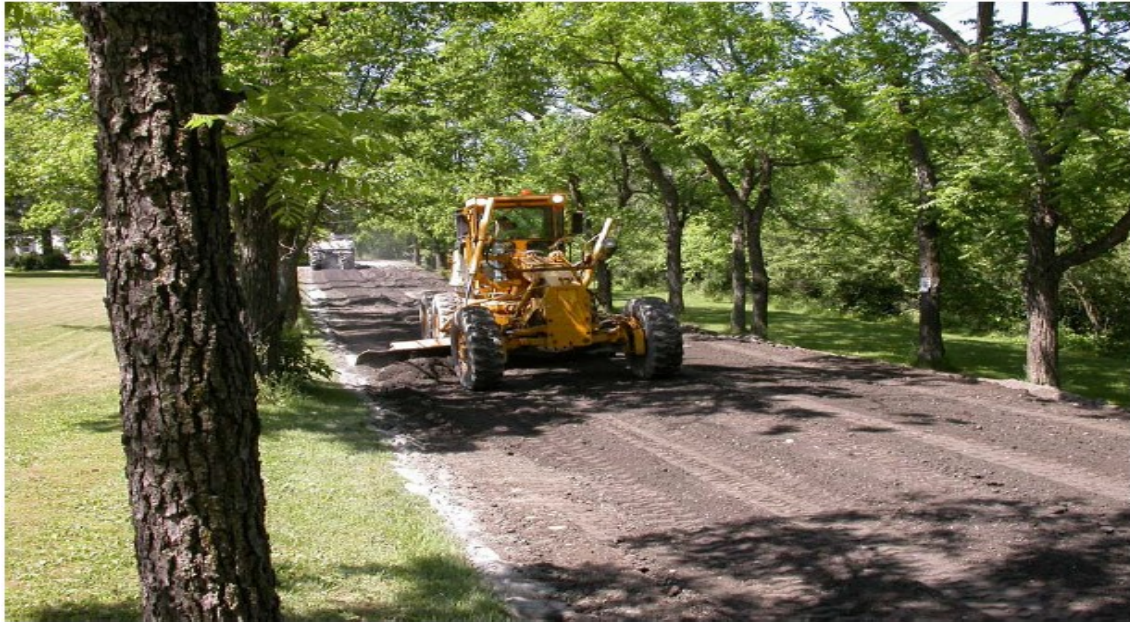
Figure 2-4 Shaping the pavement with a grader (Morian et al., 2012)
