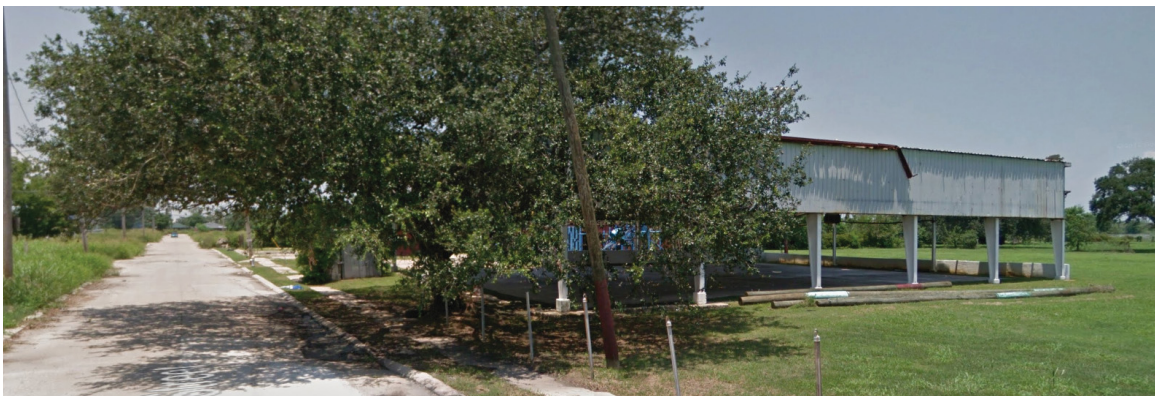
Images of the derelict portal frame structure (Google Maps 2014)
