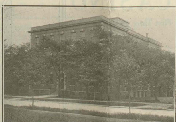
PATHOLOGICAL BUILDING. Photo by MacAskill.
