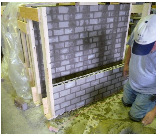
a) First stage of construction
