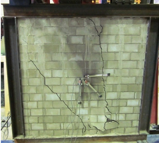
c) Additional cracks in specimen 4
