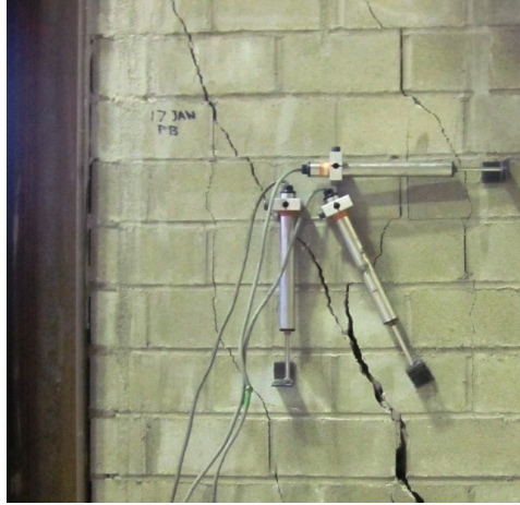
Figure 4.29. Cracks developed across the length of LVDTs
