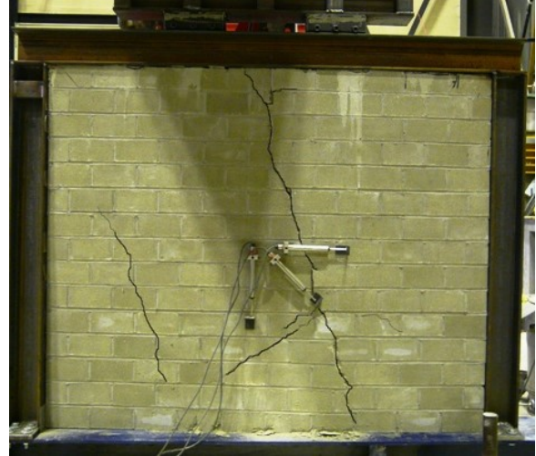
d) Additional cracks in specimen 5
