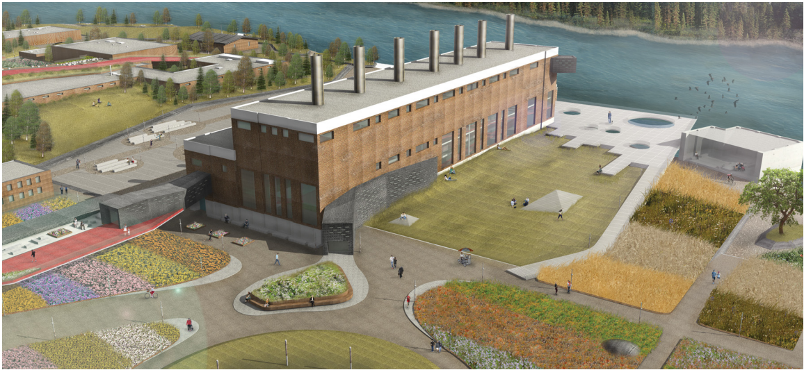
Fig. 28. Bird's Eye Perspective of the Rosedale Generating Station.
