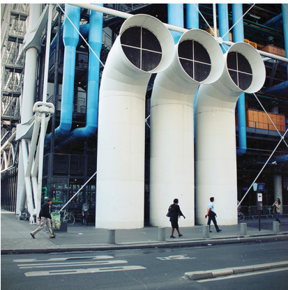
Centre Pompidou's exposed ductwork (Vitamean 2012)
