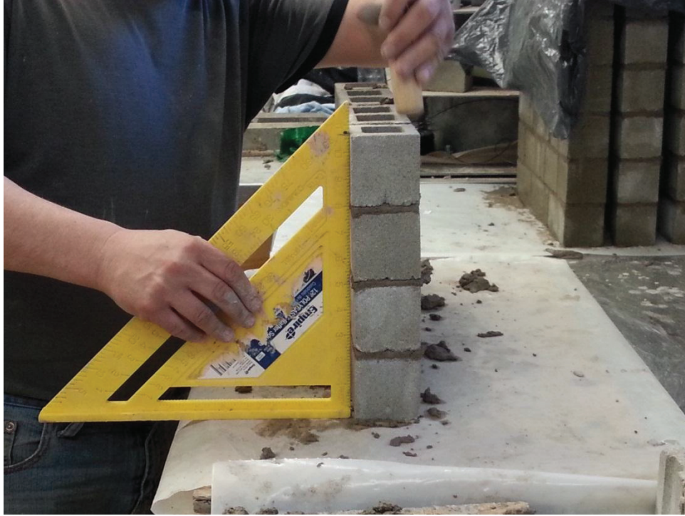
Figure 3.10 Leveling the concrete blocks during placement
