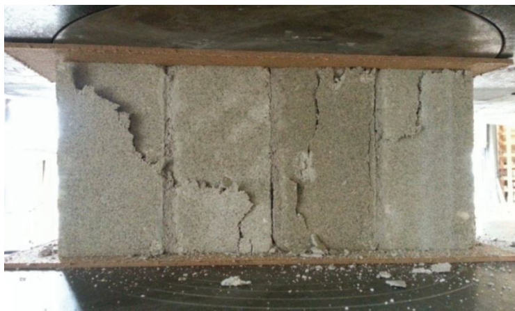
Vertical Crack (face-shell)
