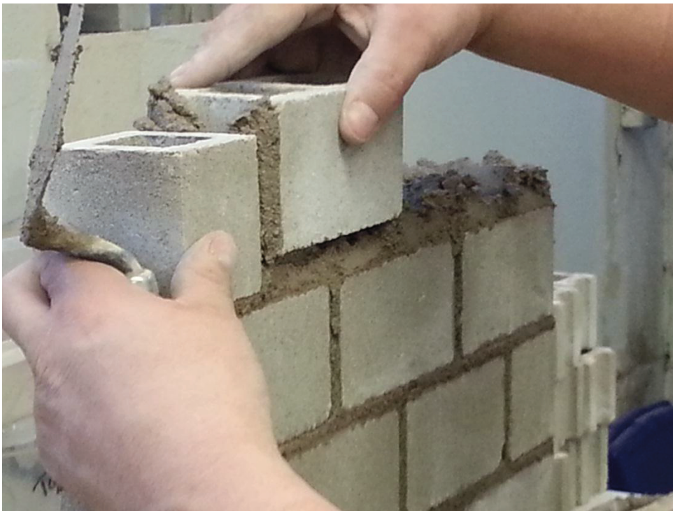
Figure 3.11 Mortar Placement
