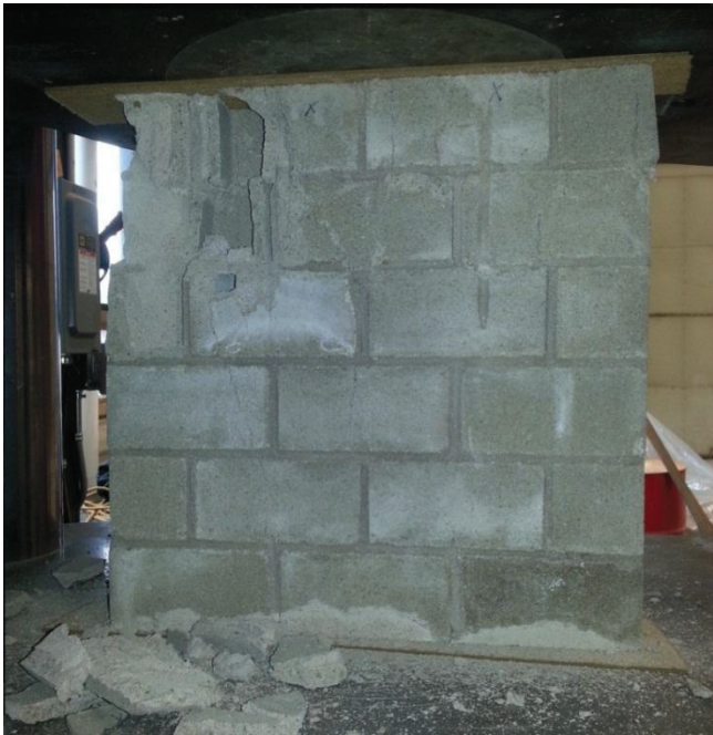
Figure 4.23 Failure mode of specimen S2- PNV
