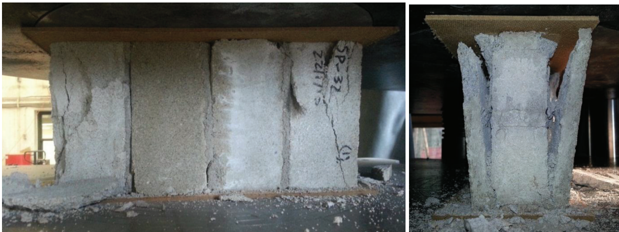
Figure 4.15 Failure mode of specimen S1-F4NH
