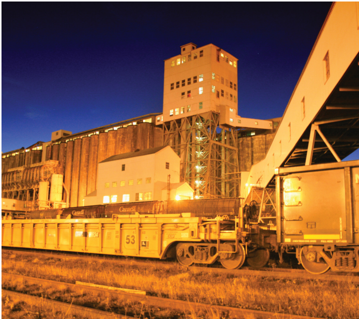
Photograph of grain elevators at night.
