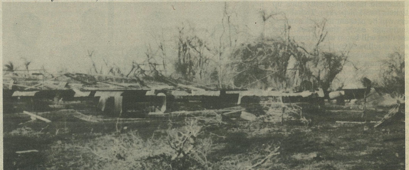
This is what remains of a poultry house which held 17,000 laying hens. The farmer gave away the birds that survived and burned the dead ones. All types of animal shelters were extensively damaged and the cost of rebuilding is a great burden for many small farmers.
