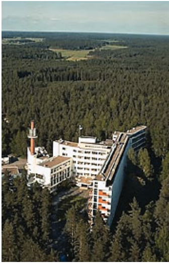
Paimio Sanatorium by Alvar Aalto showing the surrounding forest, from Nakamura, Alvar Aalto
