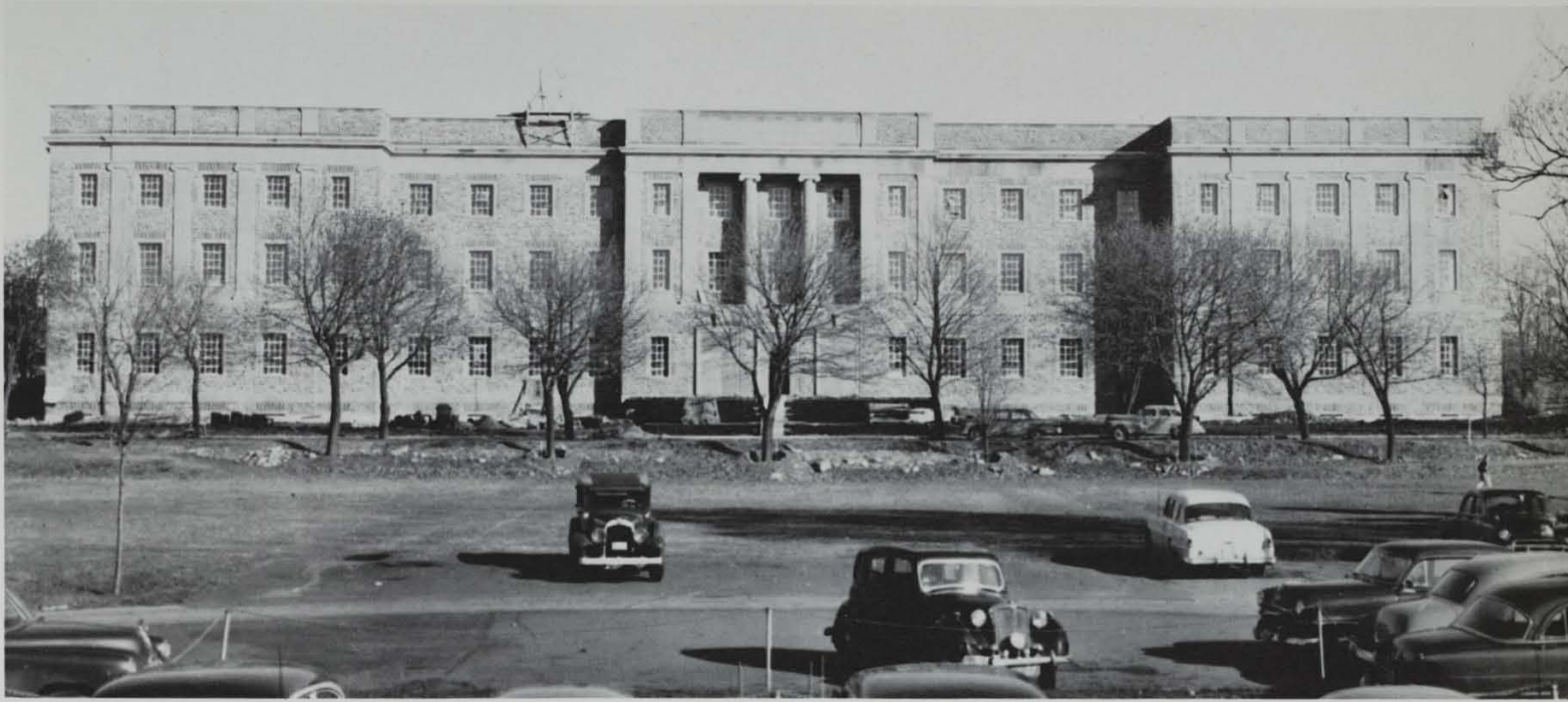
Shown above is construction on the Sir James Dunn Science Building in the early 1960's. It was a gift of the Sir James Dunn Foundation.
