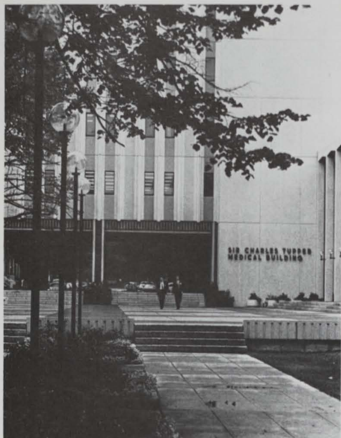
Sir Charles Tupper Medical Building — Dalhousie.
