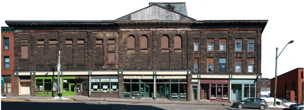
Current condition of Wood Block building - south elevation
