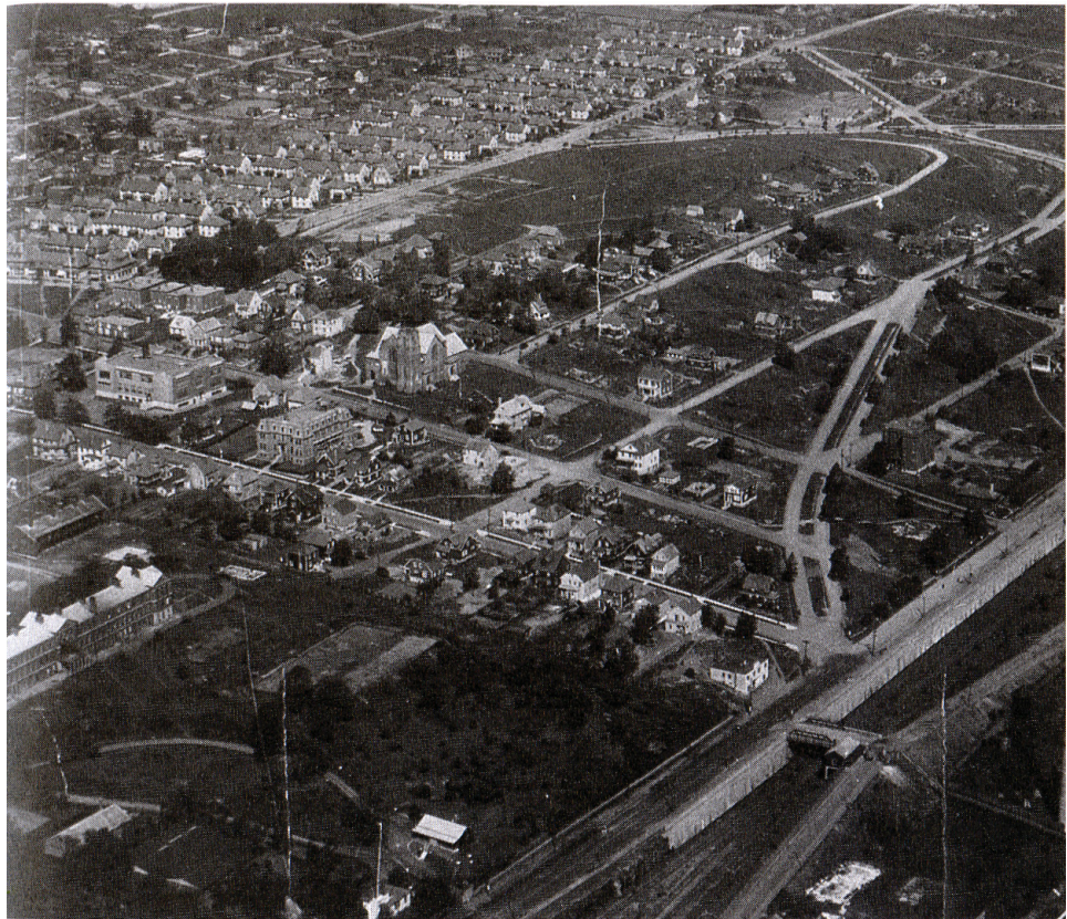
Rebuilt Former Richmond with the newly built homes of the Hydrostone district clearly seen at the top right (1930).
