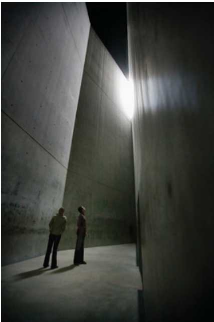
Rooms within the Jewish Museum: The Garden of Exile and Emigration; Holocaust Tower. Berlin, Germany. Source: Daniel Libeskind Studio .
