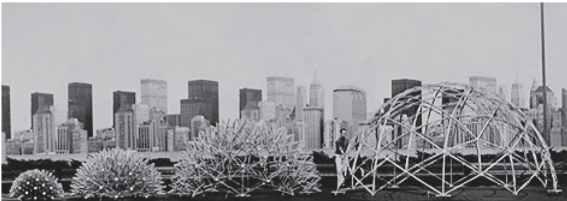
A sequential image of the erection Hoberman's expanding geodesic dome, 1991 (Hoberman Associates 2012).
