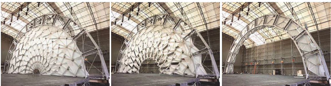
Opening sequence of the Hoberman Arch. The deployment is accomplished by the arch acting as a stable base that the kinetic units are attached ( CrossLab Yuki Blog 2012 ).
