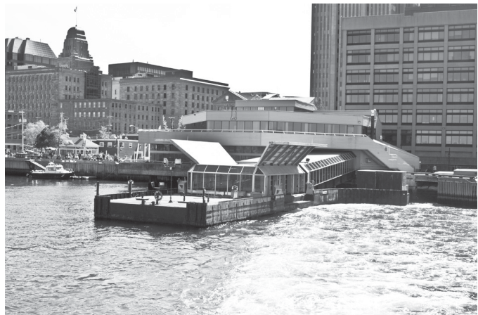
Current Halifax Ferry Terminal
