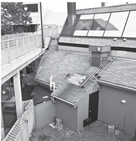
Leftover space behind Murphy's on the water. Picture taken from the roof of the Halifax Law Courts.
