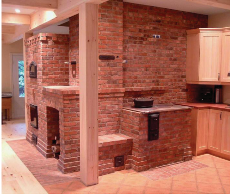
Example of a masonry hearth accessible from more than one side. From De Decker, 2008.
