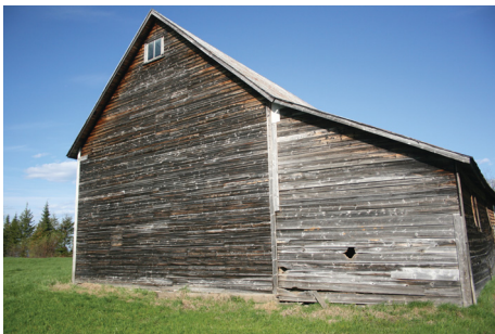
Typical abandoned maritime barn.
