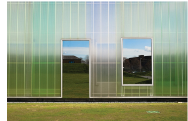
The translucent facade made from polycarbonate panels. Image from Trinity Laban.
