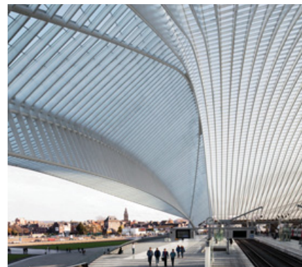
Vaulting Canopy - Liège Guillemins Station. From Minutillo, “Liège-Guillemins TGV Railway Station.”
