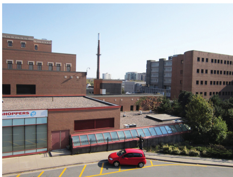
View of existing Halifax Infirmary buildings from the parking garage.
