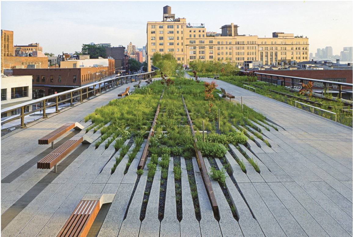
The High Line, Diller Scofidio+Renfro and James Corner Field Operations, New York City, USA. From Duran and Herrero, The Sourcebook of Contemporary Green Architecture .
