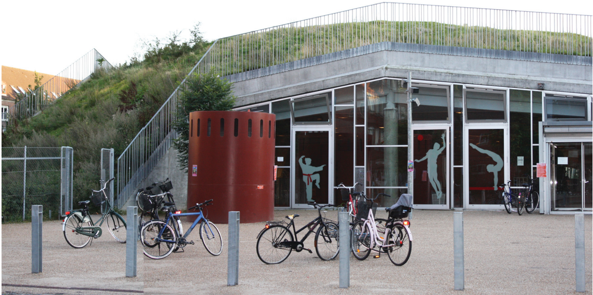
Korsgadehallen Sports and Cultural Centre, designed by BBP Arkitekter, Copenhagen, Denmark.
