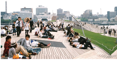
Fig. 44 The roof of the Yokohama Port Terminal by FOA uses wood to provide a hard landscape, that still invites people to sit and lounge (TKY - JP 2010).
