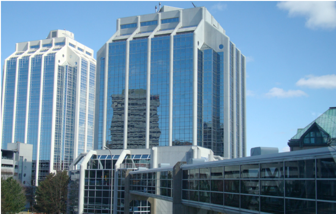
Figure 1.2: The glass covered Purdy's Wharf towers in Halifax are part of the city's identity.
