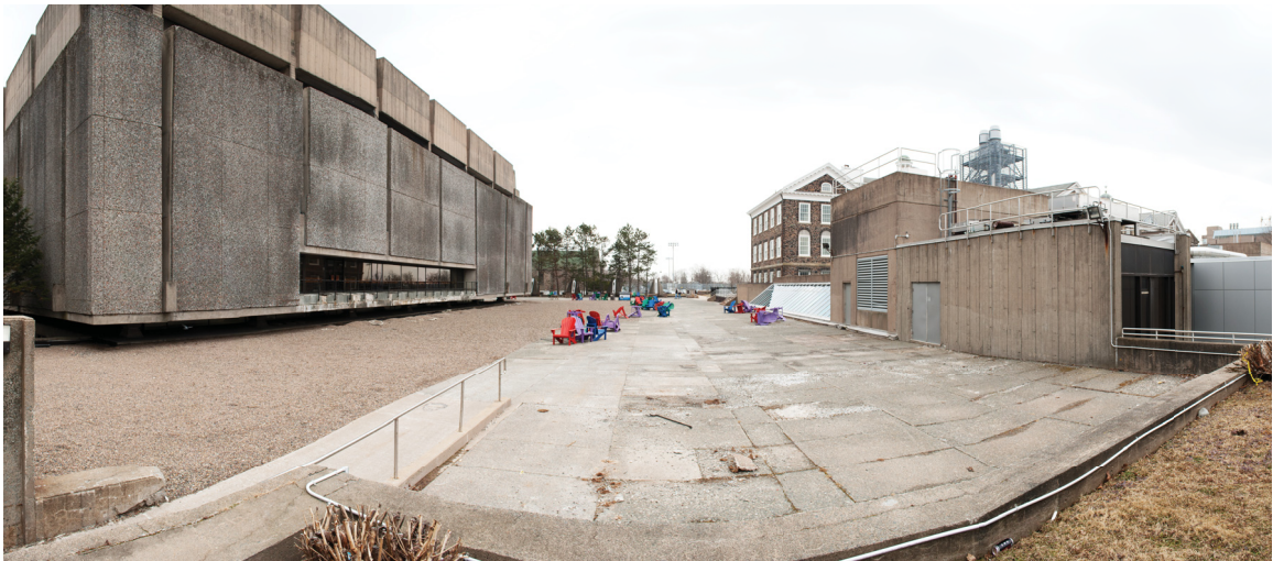
Site looking south.
