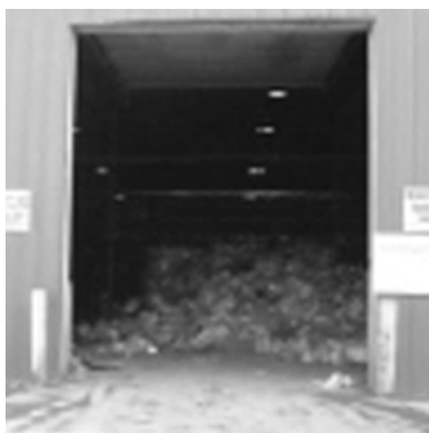
Typical waste management facility - tipping floor.
