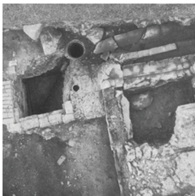
Stone sewer, typical in the 1800s. (Erickson 2005, 16)
