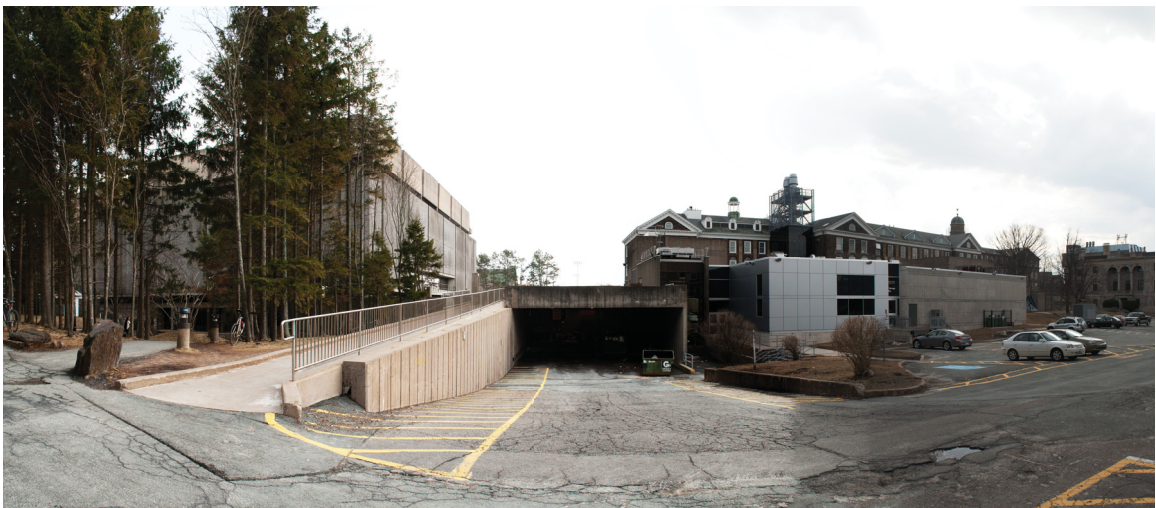
Site looking south at loading dock.
