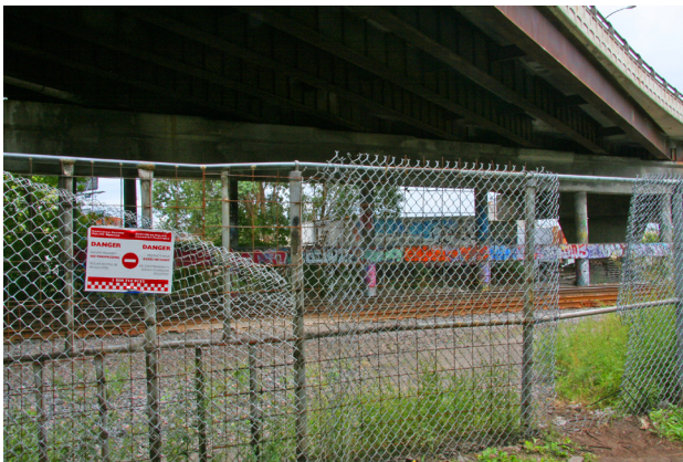
The direct cross way ramp will border the viaduct.
