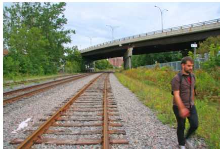
The viaduct over the railway
