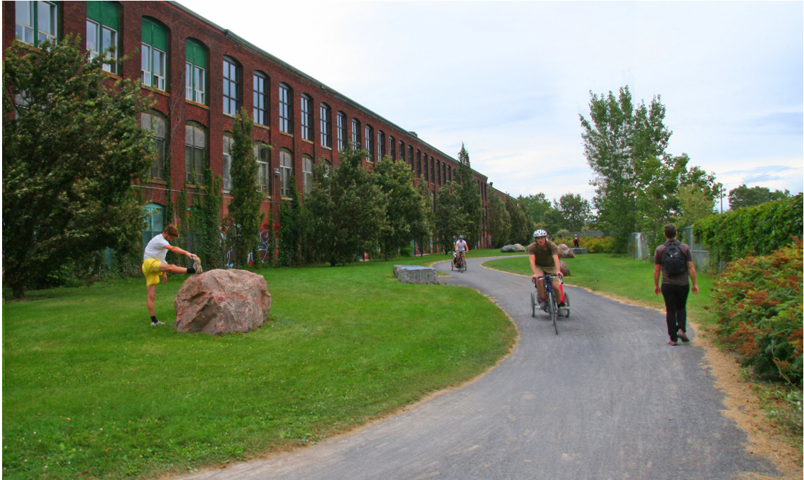
The numerous bikers and joggers that use the bike path rarely use the viaduct to cross the railway.
