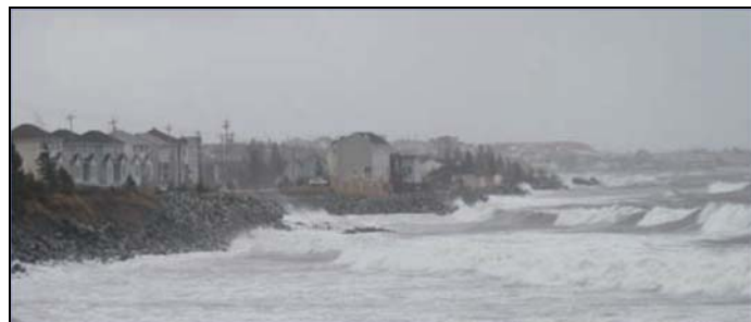
Figure 4. Large rocks were placed along the shoreline to protect these homes along Halifax Harbour from storm damage.
