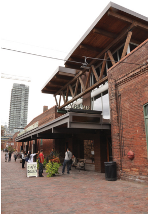
Young Centre for the Performance Arts. Main Lobby space was created by straddling two existing buildings to allow infill between the two buildings.
