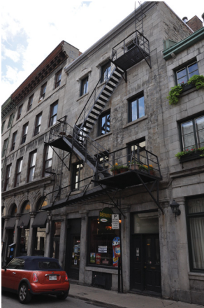
Montreal. Photo of fire stairs being used as balconies.
