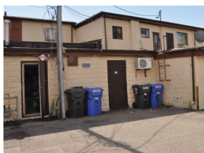
Diplock Lane. Programs in the back end of the buildings is used for storage.
