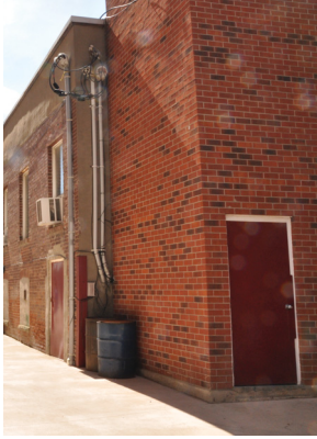
Harmsworth Lane. Electrical cables attached to exterior facades.
