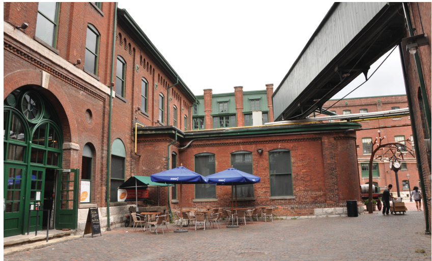
Exterior Patio. View of cafe utilizing void space as patio.
