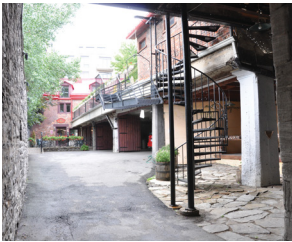
Montreal. Cafe extends out into area that is also used for parking along the side.
