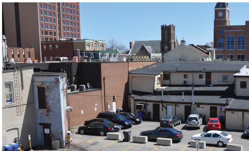
View looking at existing condition of site.
