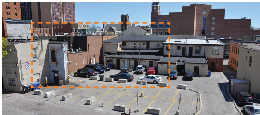
Diplock Lane. Looking south toward site highlighted in orange.
