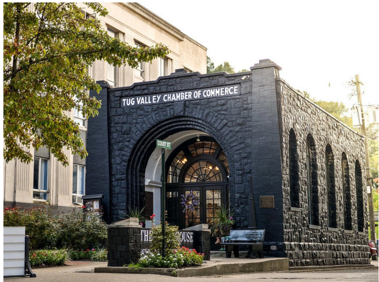
The front facade of the West Virginia Coal House, clad in locally mined coal (Graham 2018)
