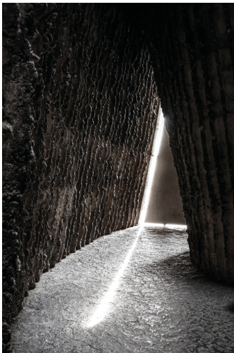
The interior cavity of P. Zumthor's Bruder Klaus Field Chapel in Eifel (2007) is formed from burning 112 tree trunks (Sveiven 2011)
