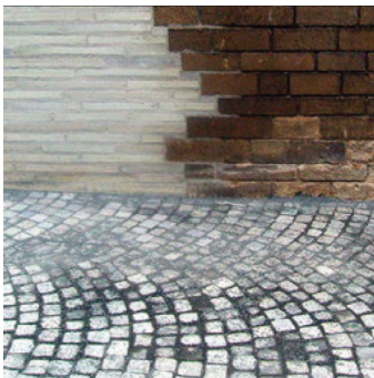
Kolumba Museum detail of Zumthor choosing to accentuate differences with the new brick rather than mimic the old (Goffi 2016, 32).
