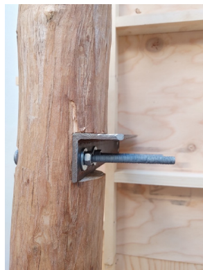
Connecting the steel fastener
