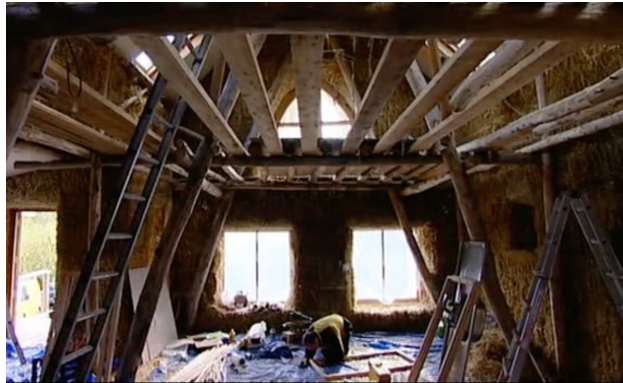
Straw bale insulation on the interior eliminating any expression of the stud wall. Still from video (Law 2015).
