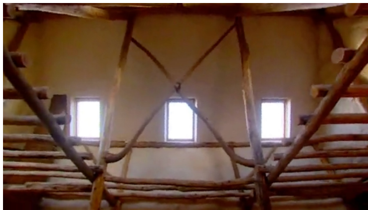
Cross bracing utilizing the sweep of the two trees (Law 2022)
