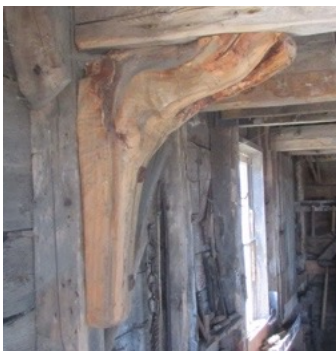
Ship's knee. Interior of the 'Reuben Tefry Blacksmith shop,' Le Village Historique Acadien. Photograph: David Goldsmith
