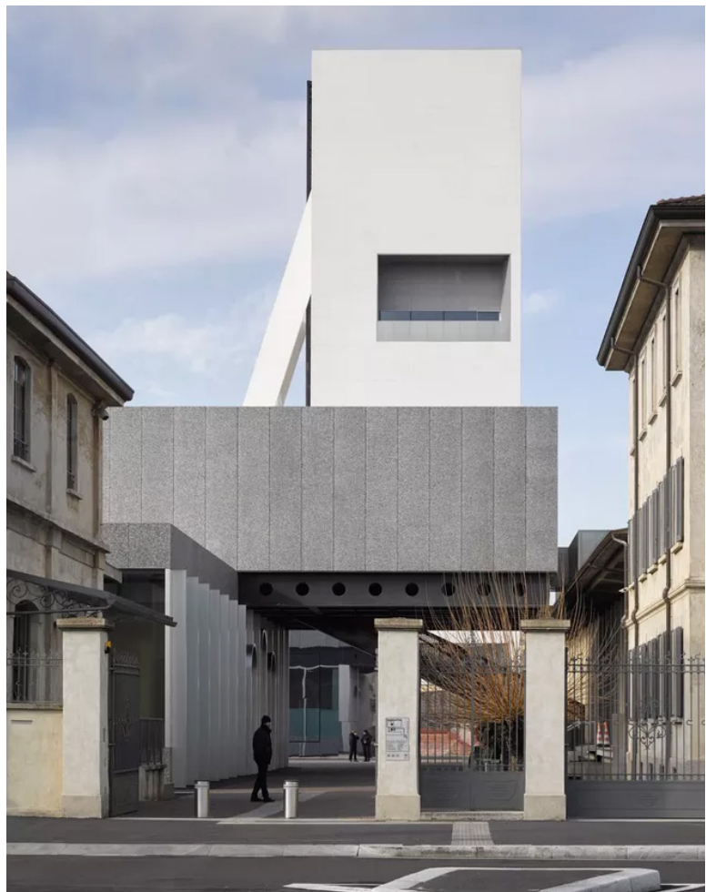
The Prada Foundation's exposed structure (OMA 2018)
