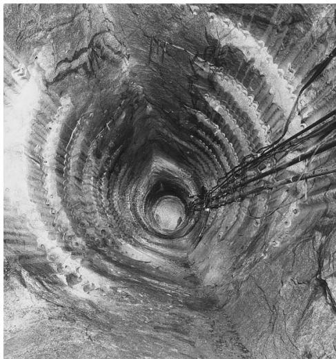
Figure 1-1 An example of v-shaped notch failure around a circular test tunnel at the URL (after Read et al., 1998)
