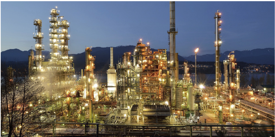
Chevron oil refinery at night. Burnaby, British Columbia. (Oil Sands Magazine 2019)
