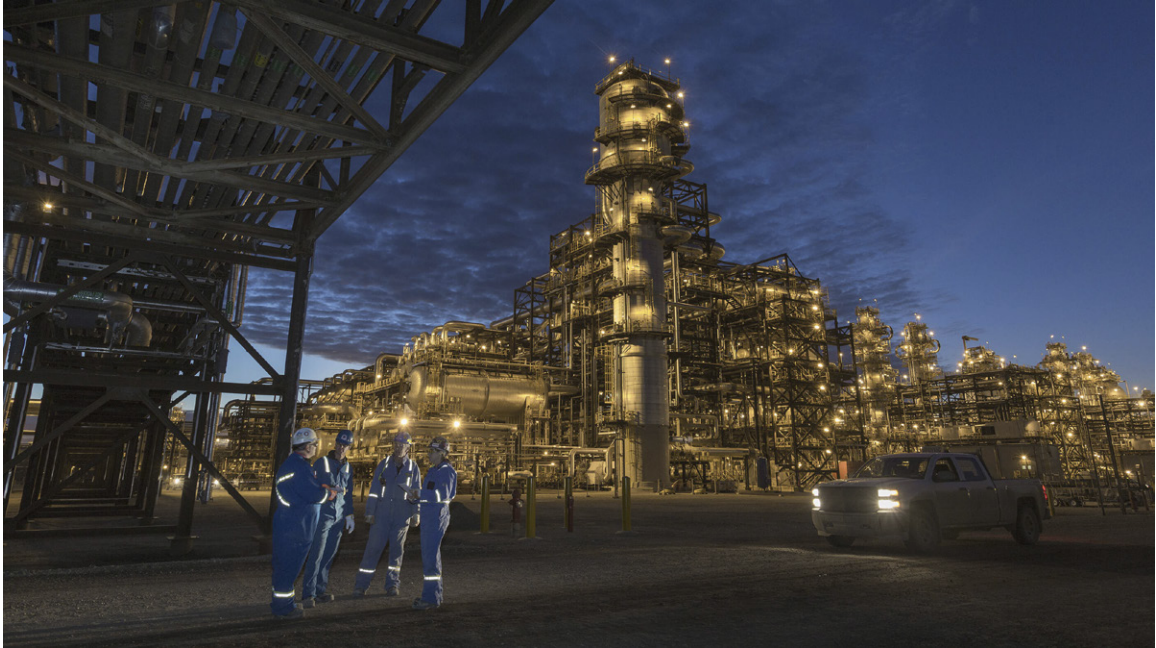
Object of attraction: Infrastructural attractor and elevated piperail structure. Oil refinery at night. (Imperial Oil Limited, 2019)
