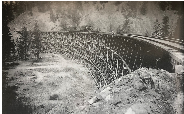
765-foot long wooden frame trestle built from the surrounding forest, 1920; photo courtesy Andrew McCulloch Foundation (Sanford 2010, 96)
