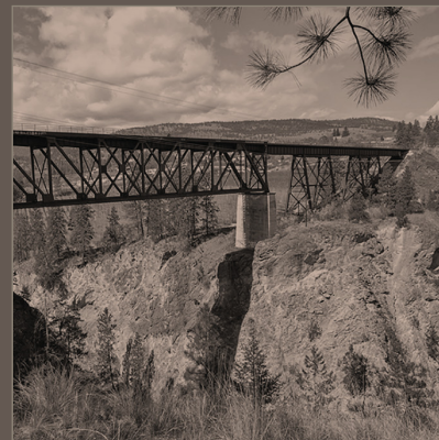
4 TROUT CREEK BRIDGE
