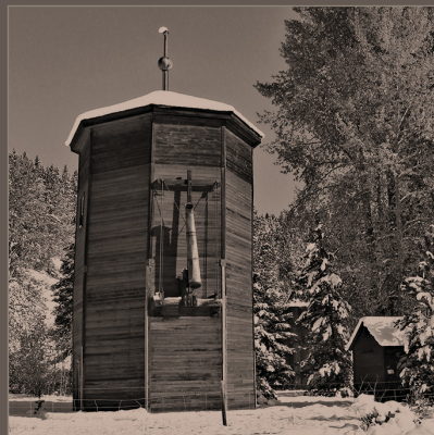
3 BROOKMERE WATER TOWER
