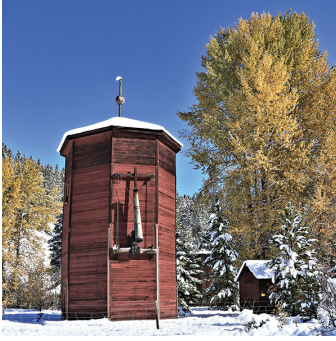
Brookmere Water Tower - the only water tower along the KVR that has not been reduced to a foundation, n.d.; photo courtesy Doug Smith (Smith 2019)
