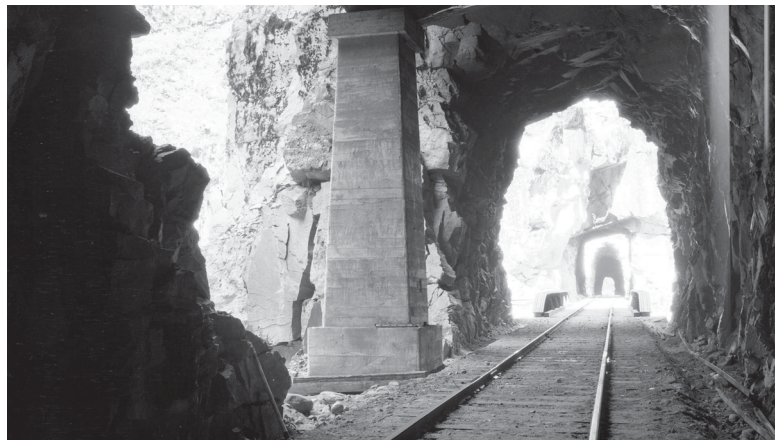
Piercing the granite canyon walls, Othello Tunnels creates a perfect tangent alignment through the landscape; photo courtesy Andrew McCulloch Foundation (Sanford 2010, 96)
