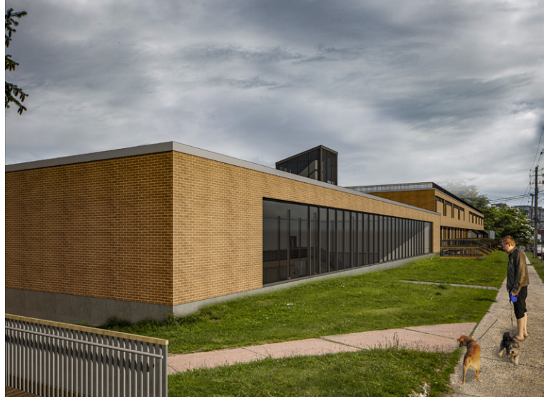
Maitland Street view of work shop (3 in plan)
