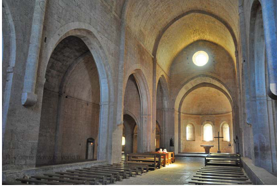
The church at the monastery is designed for Gregorian Chant. There is a 14 second reverberation time, perfect for acapella singing in unison. Photo by Stan Parry, "Nave and Apse," in Stan Parry Photography Art and Architecture Photography .
