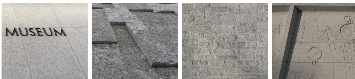
Image 39 [From left to right] Clean cut Tyndall stone, rusticated Tyndall Stone, uncoursed square rubble Tyndall stone, and petroglyphs on Tyndall stone
