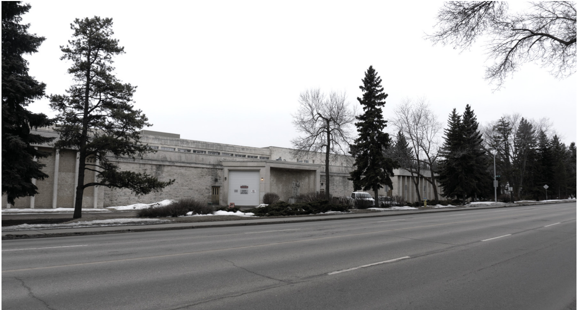
Image 70 Existing monolithic North elevation
