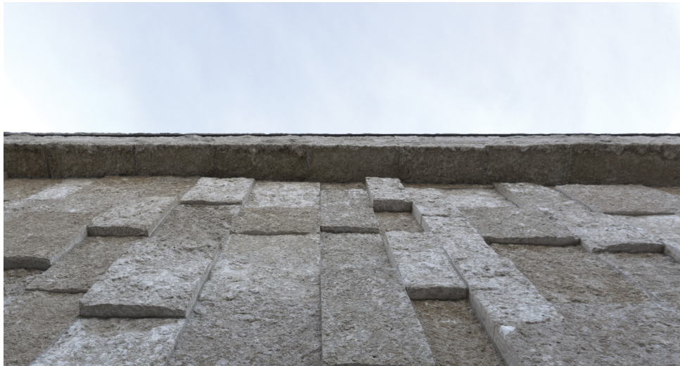
Image 49 Rusticated Tyndall stone from archives building
