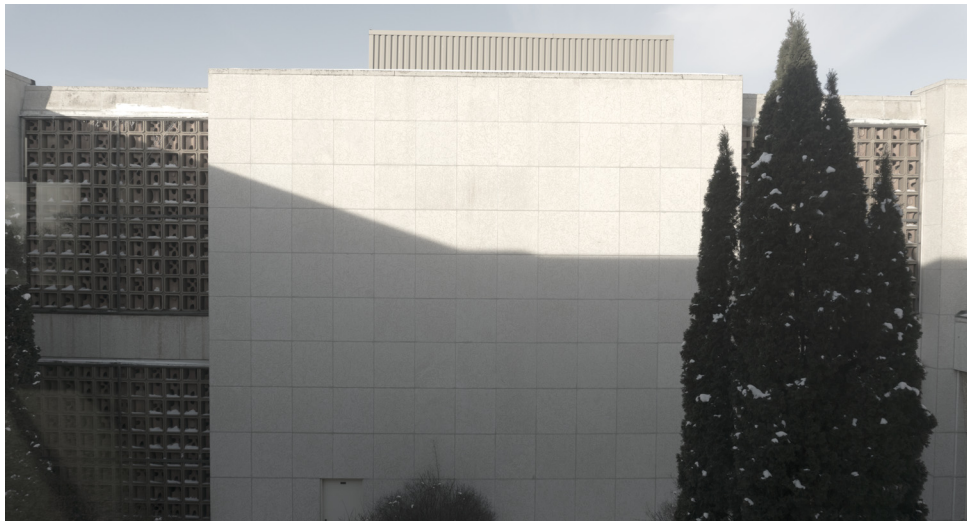
Image 50 Clay architectural screen in courtyard
