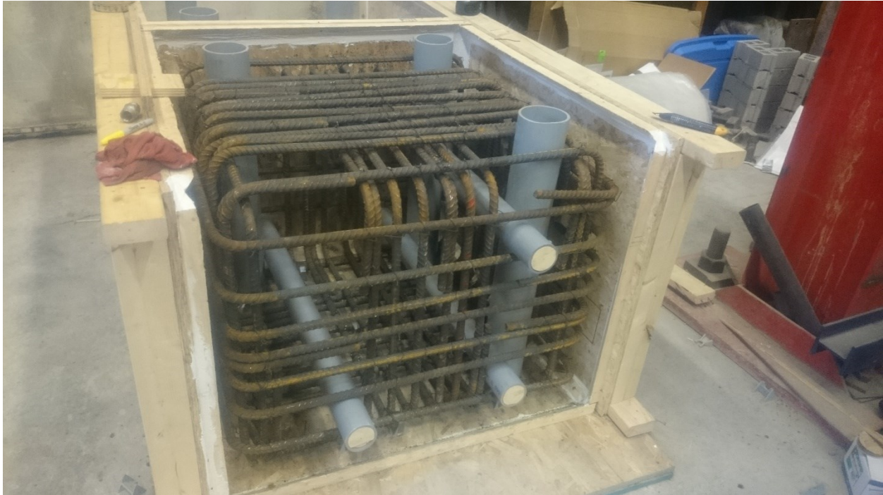
Figure 24: The internal reinforcement of the end block with the PVC tubes for the internal voids to secure samples to the block and the block to the floor. Note: at this point, one of each type is missing but was later added in.
