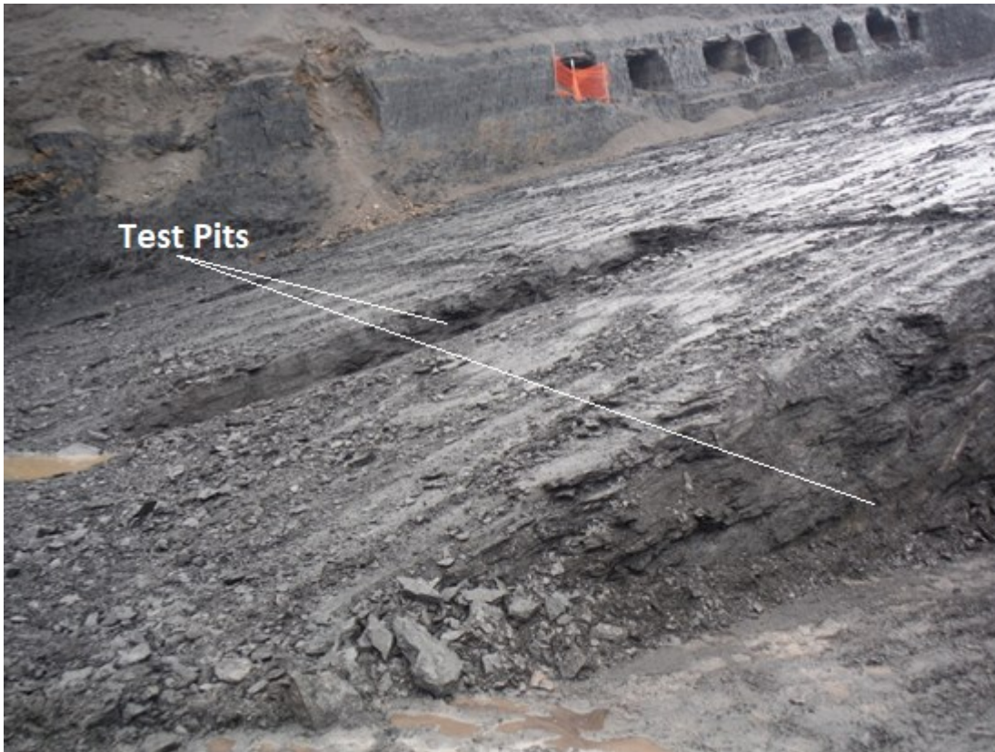
Figure 48: Image of the test sites in the coal/shale mix.
