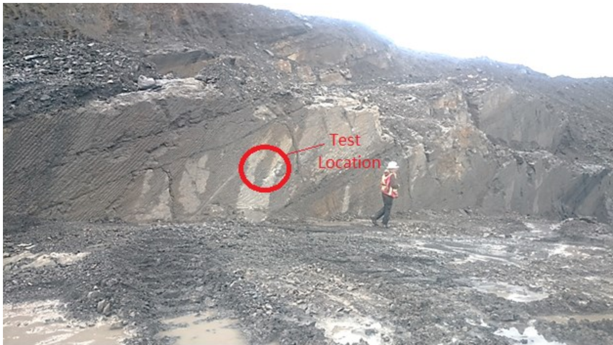
Figure 52: The wall test location. The cut was made directly behind where the engineer is standing.
