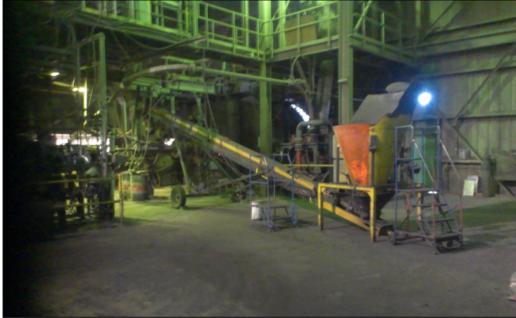
Figure 35. Improved hopper and conveyor assembly for delivering shingles as received.
