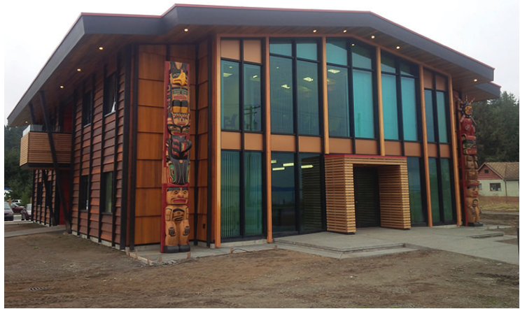
Integration of traditional native methods; primarily cedar siding over post-and-beam framing (Wedler Engineering 2015)
