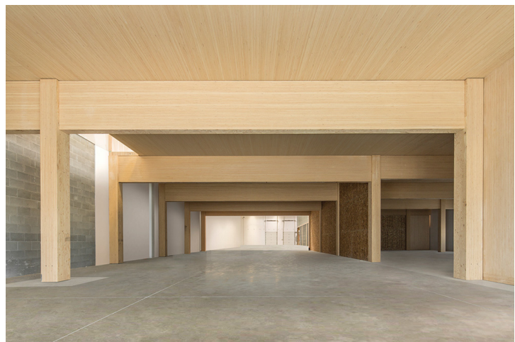
Engineered CLT shear diaphragm and post-and-beam (Green 2015)
