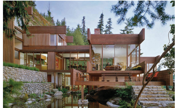
Anchor, transition, and pile ground connections navigate a dynamic topography (Erickson 2015)
