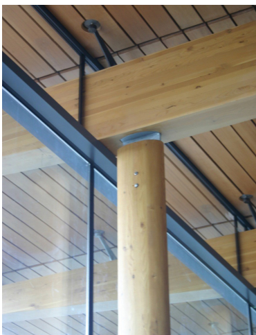
Steel jointed post-and-beam (Green 2015)
