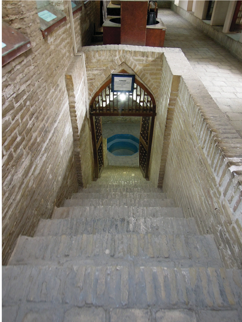
A traditional Persian home uses the water from a qanat to temper the air. This is an example of an inhabitation of a building system. Yazd, Iran, 2014. Photo courtesy of Hamid Mohammadi.
