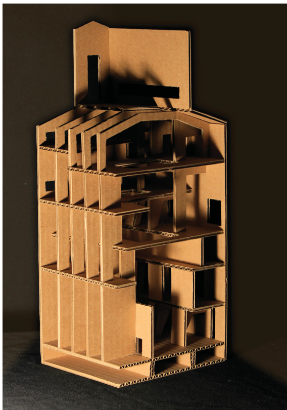
A spatial study of a wooden grain elevator that measures 115' tall (90' shoulders). Bin capacity: 70 and 110 tons. Original model scale: 1:100.
