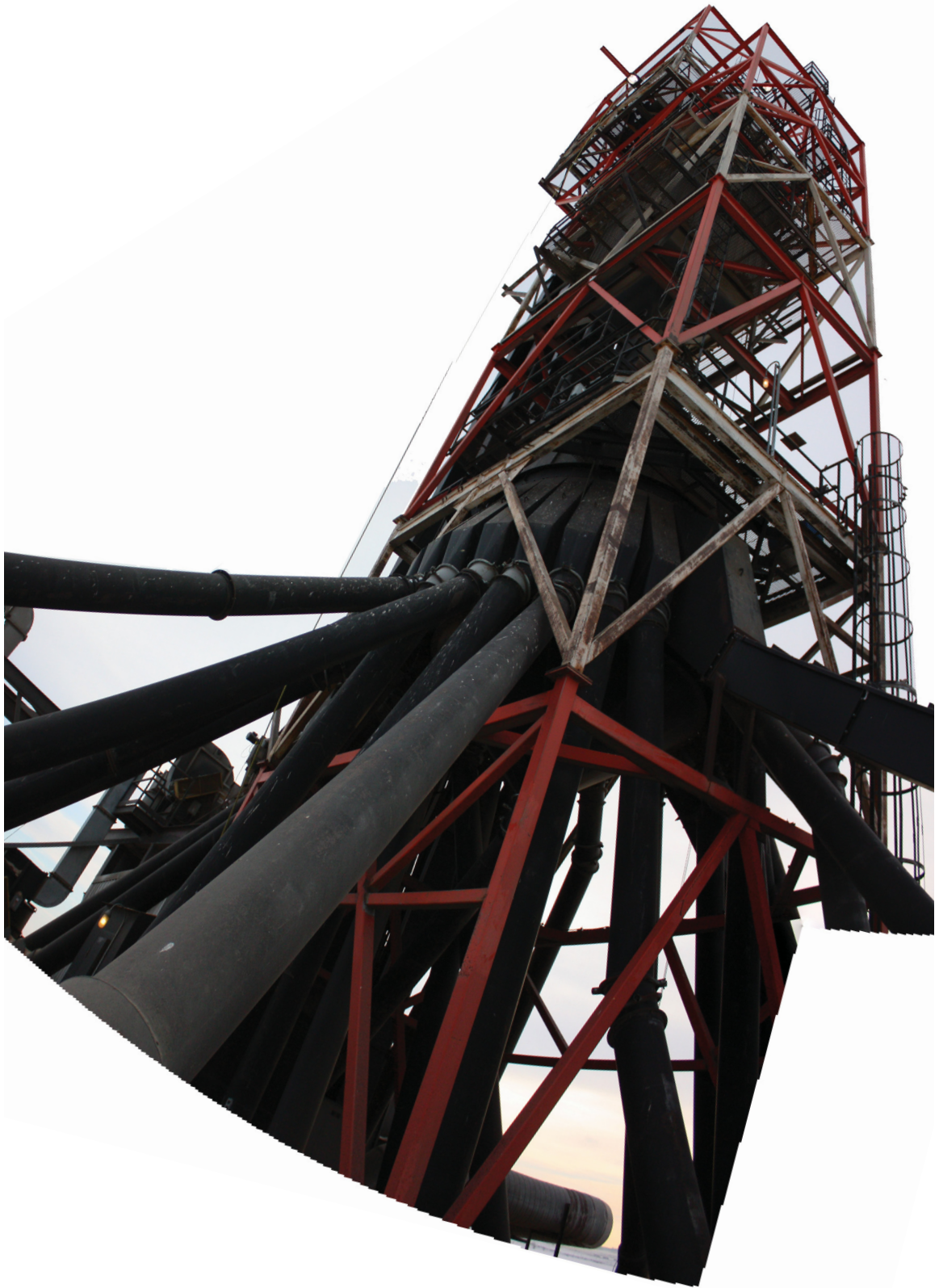
A representation of the steel structure and grain flow above concrete silos.
