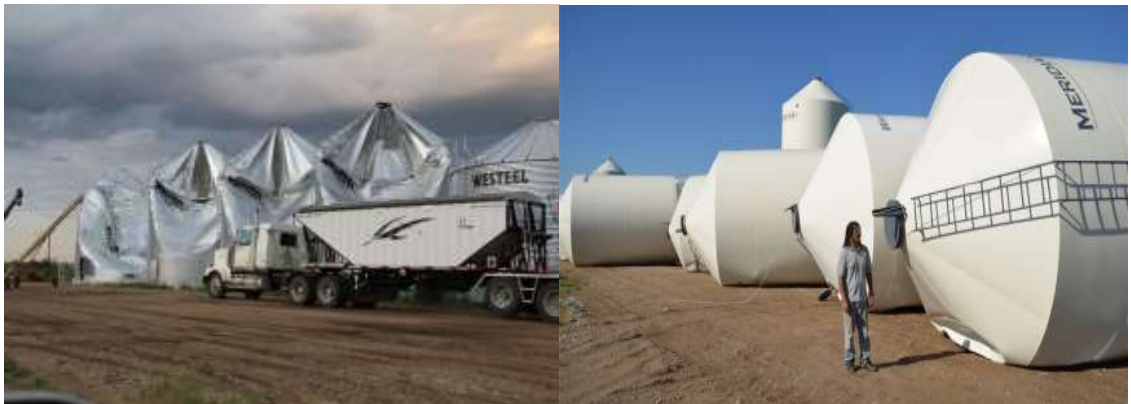
Figure 4.16 Plow wind damage. Source: www.northernprideml.com
