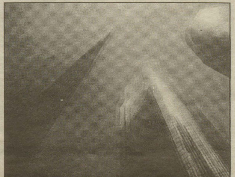
These buildings should be fixed cause they move around a lot.
