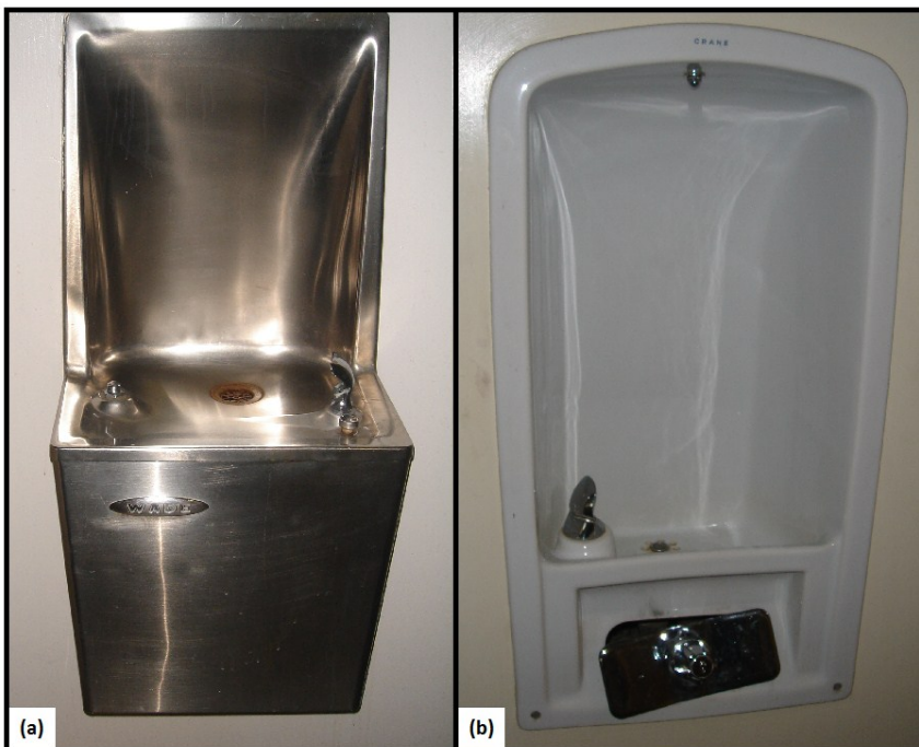
Figure 4.1: The fountains at the focus of this study (a) Halsey Taylor RWM model and (b) Crane
