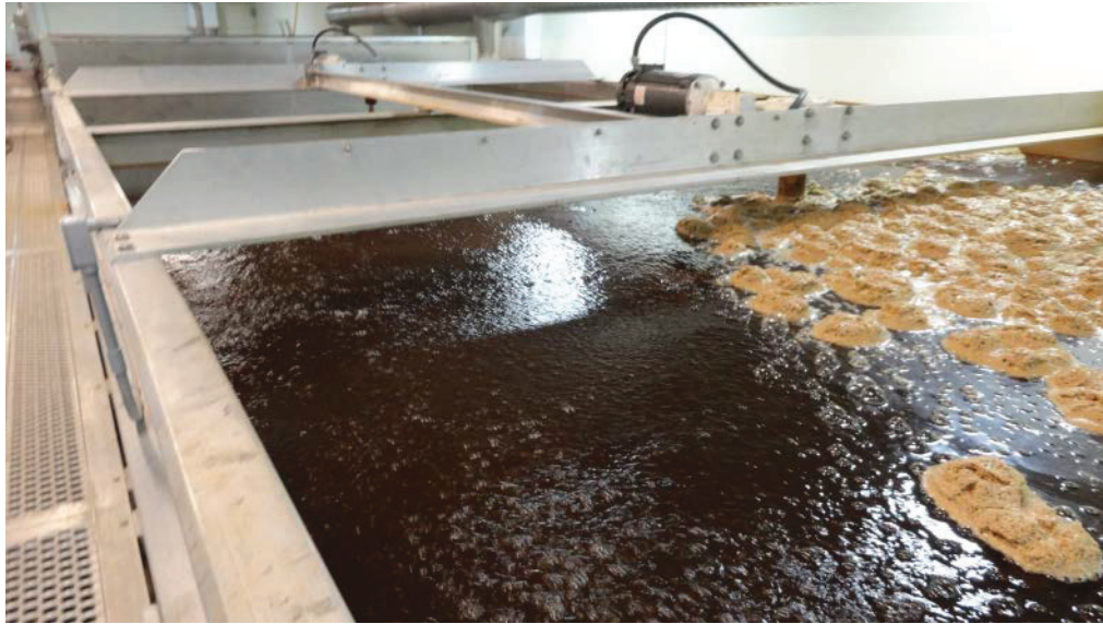
Figure 4.6. First floc basin with bubbles and surface foam.
