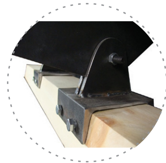
detail of steel c-channel connection
