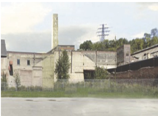
Evergreen Brickworks: Existing Conditions. Photograph (Diamond Schmitt Architects and ERA Architects 2008 a).
