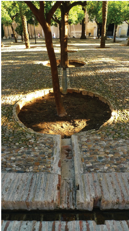
Sunken tree wells along grid that branches off main distribution channel. (Spain - Cordoba - Patio de los Narajos, Drip/Dry: Systems That Seep )
