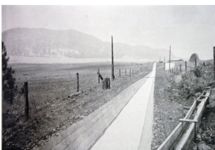
Concrete canal of Kelowna Irrigation Company with wood diversion channel to an individual lot (Rogers, Report of Proceedings of the Sixth Annual Convention of the Western Canada Irrigation Association )
