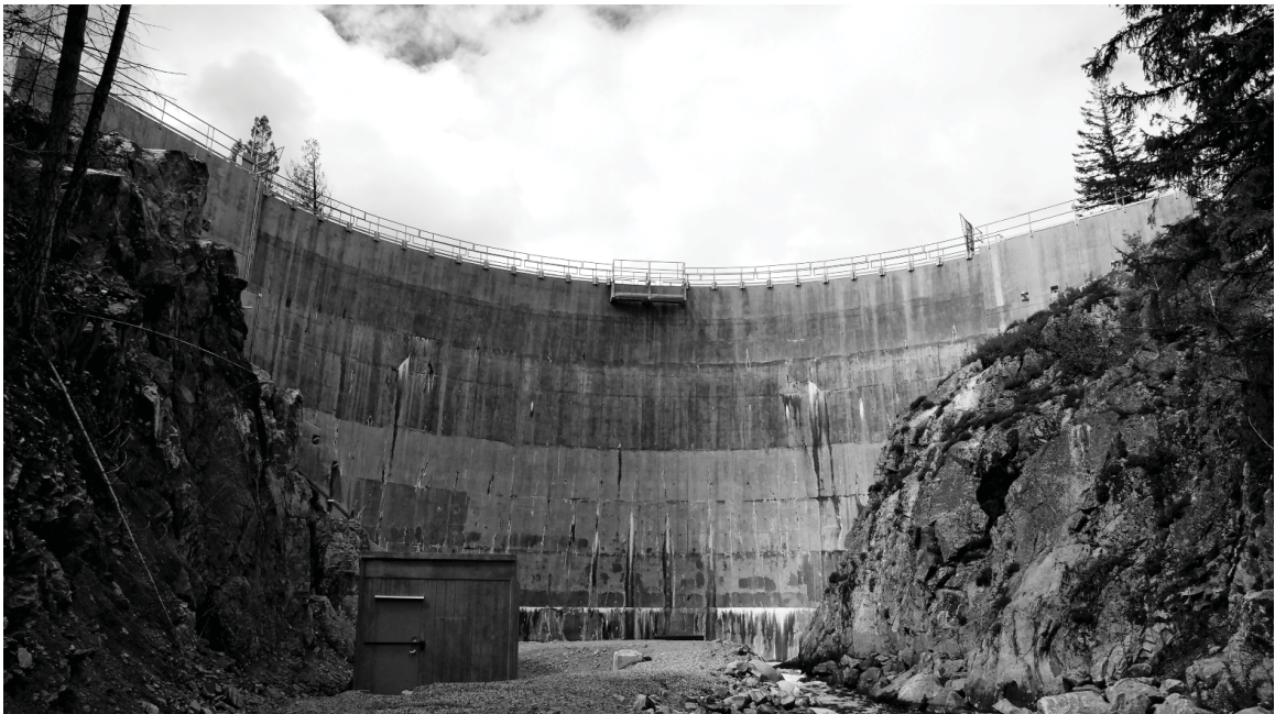
Thirsk Lake Dam as it currently stands. (Kirby, Thirsk Lake Dam ).
