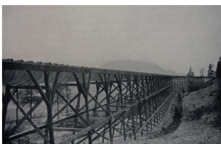
Steel flume and elaborate wooden support structure. (Rogers, Report of Proceedings of the Sixth Annual Convention of the Western Canada Irrigation Association )
