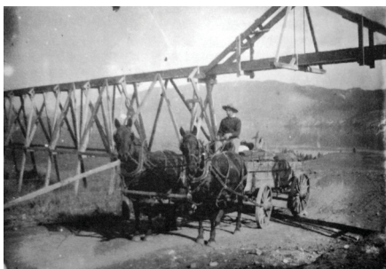
Wooden flume carrying water above roadway. This proved particularly inefficient because these structures were often damaged by wagons and motorists and the water supply would be interrupted for days while repairs were made. (Foster, According to the Giant )
