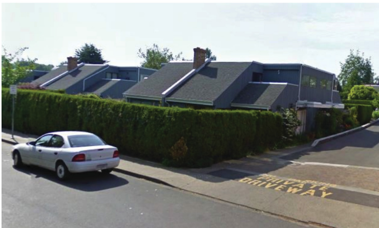
Four-plex development on the western side of the site. These buildings will be replaced.
